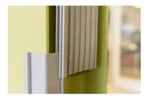
**Step #2:** To start, place the first corner panel in place and slide down the flat panel, interlocking the sections.
