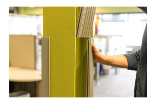
Step #4: Continue these steps by adding the next flat panel, then corner panel, and so on until the entire column is wrapped.
