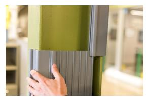
**Step #3:** Once set, add the next corner panel in place by sliding it down to interlock with the already installed flat panel.
