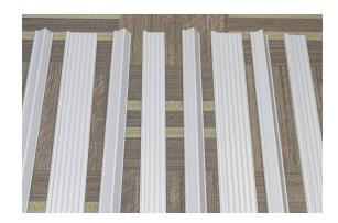
Step #1: Layout all pieces before starting installation to ensure the panel sizes and specific pieces are correct. There should be 8 pieces in total (4 corners & 4 flats).
