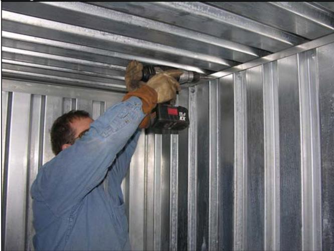
Fasten the ROOF to the front and back walls with 8pc of 1” long self-tapping screws (part no. 31806; 4 pcs. per wall). There are no predrilled holes. Space screws evenly across both walls.
