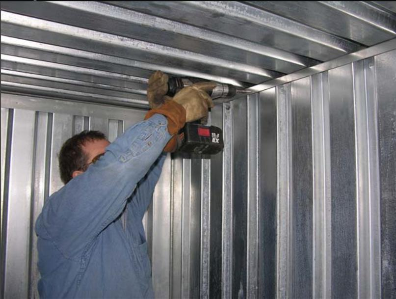
Secure roof to front and back walls with 16pc 1” long self-tapping screws (4pc per side). Holes are not predrilled. Space screws evenly.
