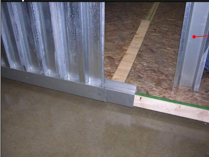
SIDE WALL CONNECTOR with concavity facing outward.
