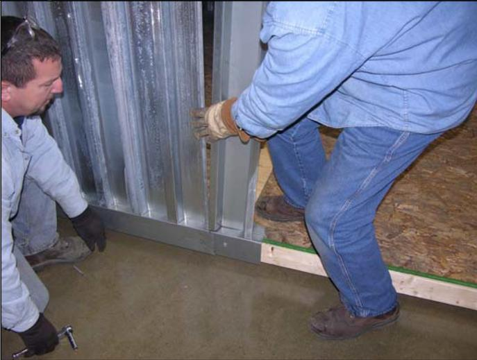
Insert the flange of one side of the SIDE WALL CONNECTOR into LOCK STRIP. Then, apply a LOCK STRIP to other flange of the SIDE WALL CONNECTOR. Repeat this step with the opposite side wall.
