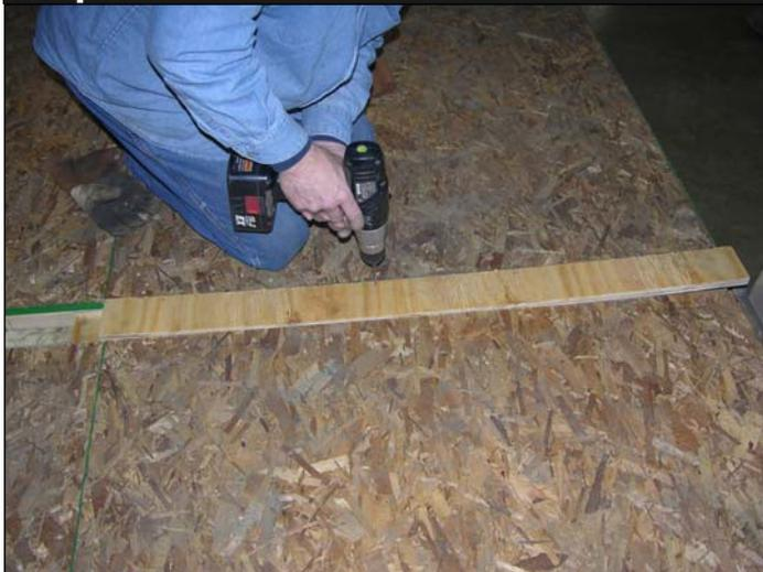
Using 20pc of 2" long wood screws fasten the plywood spacer strips directly to the 2"X4" joints. Evenly space wood screws along entire length of spacer strip. NOTE: Attach screws evenly to *both* 2x4's.
