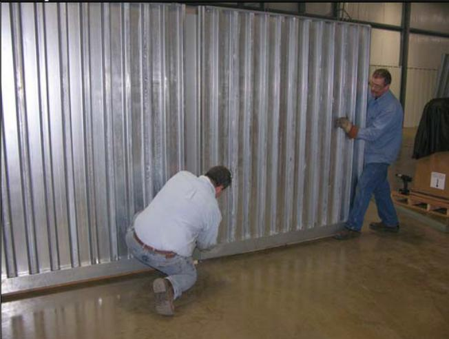
Install another SIDE WALL SUBASSEMBLY on each side. Then install 10pc 1/4"x2" lag bolts to secure walls to wooden floor. There are 5 predrilled holes at the bottom of each SIDE WALL SUBASSEMBLY.
