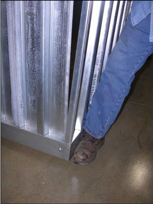
Install another SIDE WALL SUBASSEMBLY on opposite side of BACK WALL. Brace the bottom of the side wall while inserting it into LOCK STRIP.
