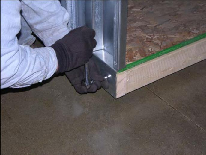
Fasten BACK WALL to the wooden floor by installing ¼"x2" lag screws (part no. 22061) through the 5 predrilled holes in the bottom flange of the BACK WALL. Continue supporting the BACK WALL until is fastened to at least 1 SIDE WALL SUBASSEMBLY this is also lagged to the wooden floor.
