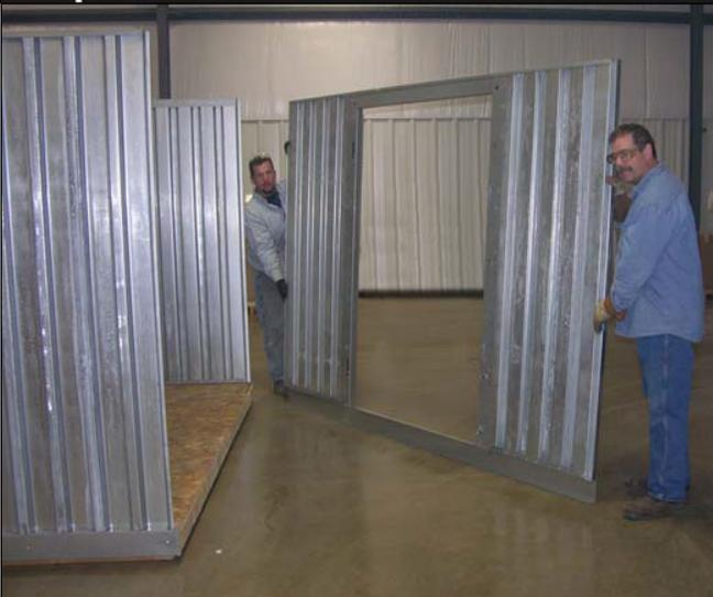
Photo shows FRONT WALL ASSEMBLY of STOR-912 without door.
