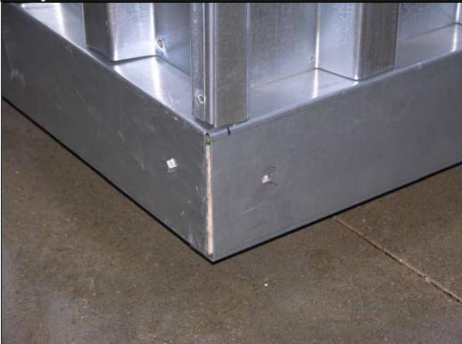
Secure both side walls to the wooden floor using 1/4" X 2" lag bolts into the 5 predrilled holes on each side.
