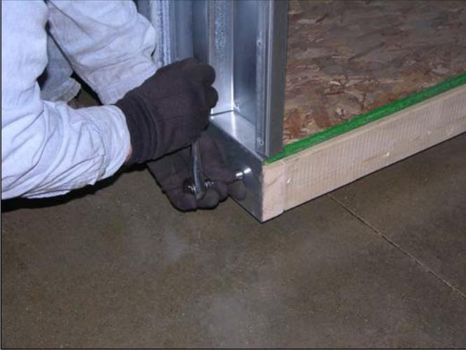
Secure BACK WALL SUBASSEMBLY to the wooden floor installing  $\frac{1}{4}$ "x 2" lag screws into the 5 predrilled holes in the bottom flange. The BACK WALL will fall over until it is attached to at least one SIDE WALL SUBASSEMBLY. Support the back wall until it is attached to at least one side wall and **both** walls are securely lagged to the wooden floor.
