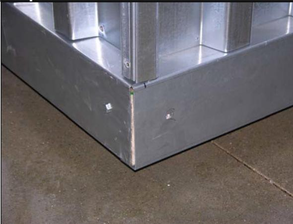
Fasten both SIDE WALLS to the wooden floor with  $\frac{1}{4}$ "x2" lag screws (22061) installed through the 5 predrilled holes in the bottom flange of each SIDE WALL.
