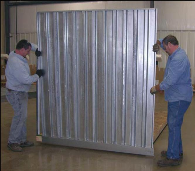
Install a SIDE WALL SUBASSEMBLY by inserting a side edge into one of the lock strips.
