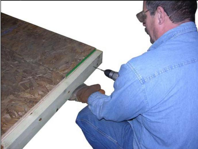
Fasten a 2"x 4" to one of the 9 foot (STOR-912) or 6ft. (STOR-612) sides of each WOOD FLOOR BASE. Attach 2x4's  $\frac{3}{4}$ " from top of floor bases (thickness of plywood) using 6pc – 3" long wood screws as evenly spaced as possible.
