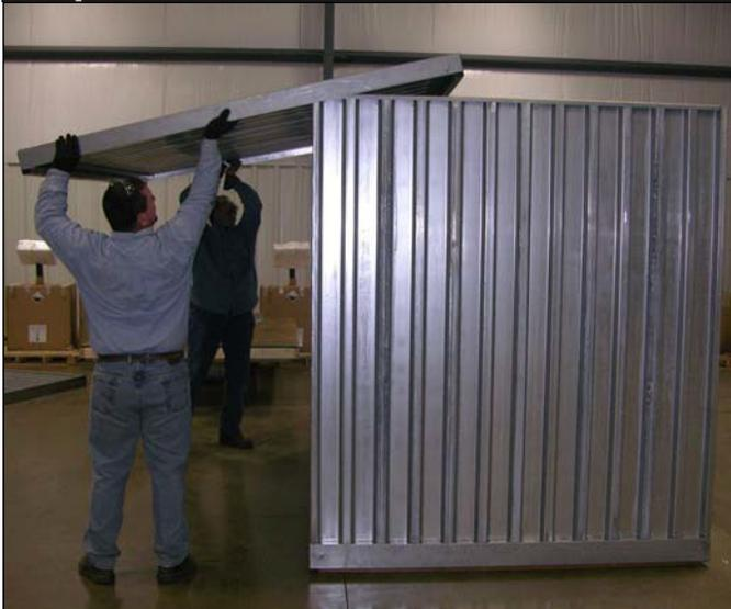
Place the ROOF WALL SUBASSEMBLY on top of the wall panels. The perimeter flange of the ROOF WALL SUBASSEMBLY must be on the outside of the wall panels. Pull/tap the ROOF WALL down until it seats onto the tops of the supporting wall panels.
