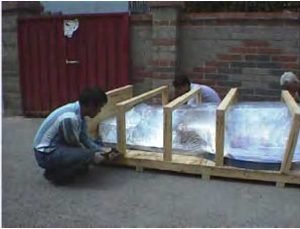
3. Fix the supporting frames.
